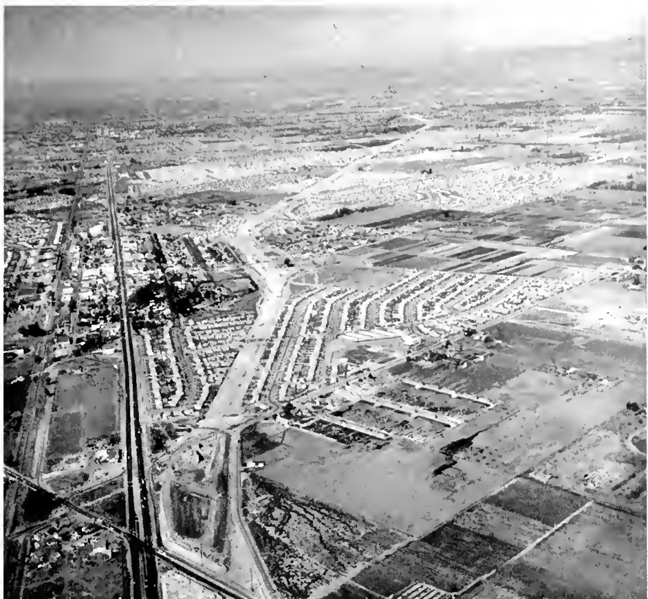
Lower Sacramento Road on Pacific Avenue extension in San Joaquin County. North end of F.A.S. project S-54312 looking south toward Stockton in the distance.
